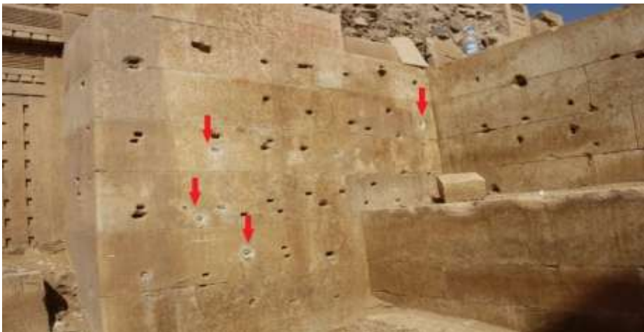
Fig. 12: Acts of tampering to the front of the internal walls of the front area foyer columns , through expanding and deepening the holes on which the votive plaques were hung, and doing other holes beside them in search of minerals (M. al-Ḥajj, 2021).
