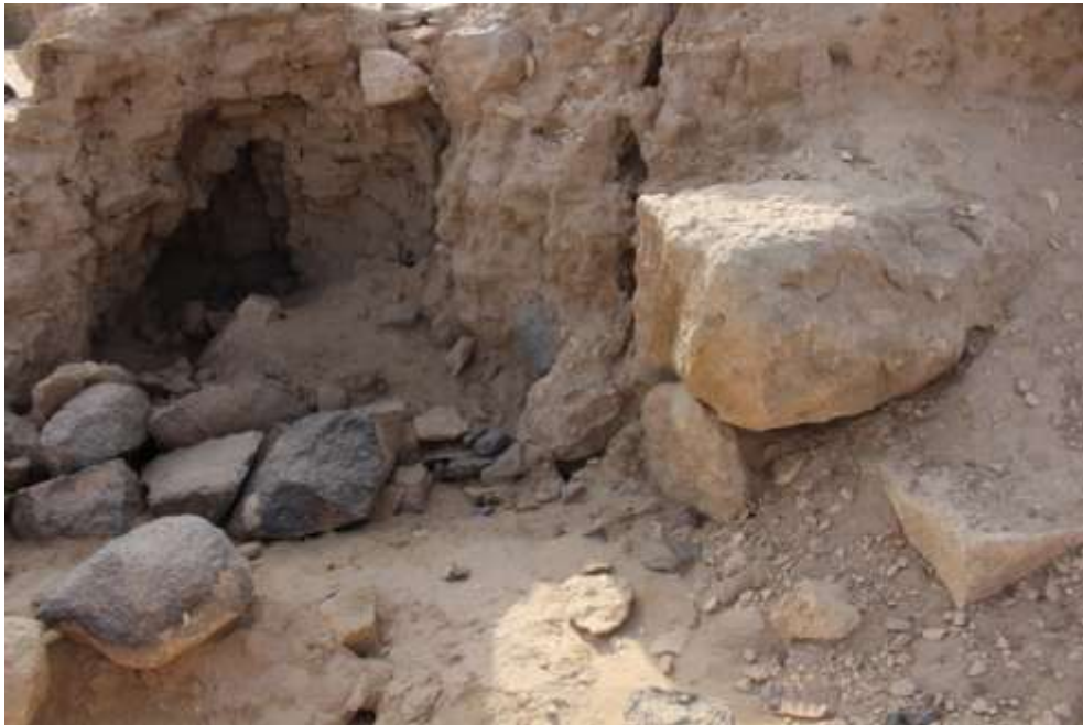
Fig. 28: the acts of digging and destruction of the diversion dam located in Ḥadiad area in Mārib Oasis (M. al-Ḥajj, 2021).
