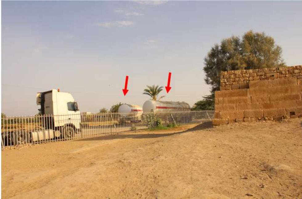
Fig. 23: storing the gas locomotives beside Bar'ān temple which causes severe risk to the survival of the temple in case such locomotives are exposed to explosion (M. al-Ḥajj, 2021).
