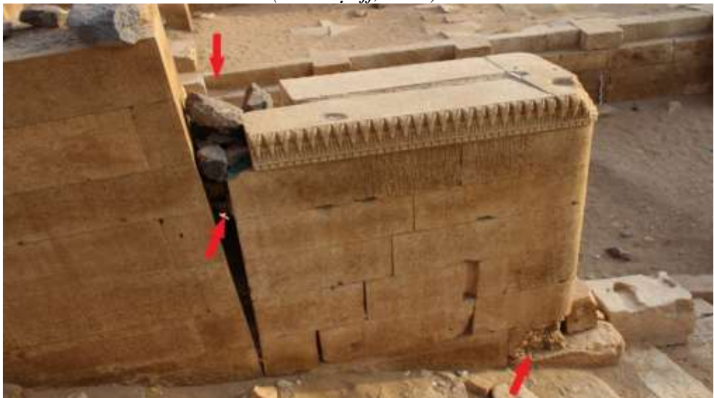
Fig. 16: the situation of the ramshackle gate of king ‘Amdān Bayyin Yuhaqbiḍ, and on its upper eaves appears the used stones in breaking it and expanding the empty place behind it (M. al-Hajj, 2021).
