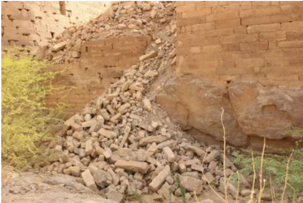
Fig. 25: the western side of the northern sluice of Mārib dam after being exposed to shelling (M. al-Ḥajj, 2021).
